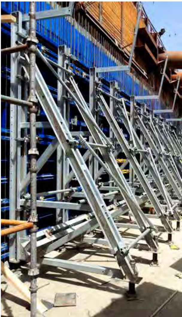
Modular supporting unit formed by combing attachable frames of 1.50 m
